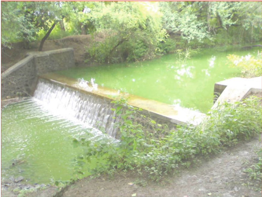
Plate 3.1 Cement nala bund at Atali village
