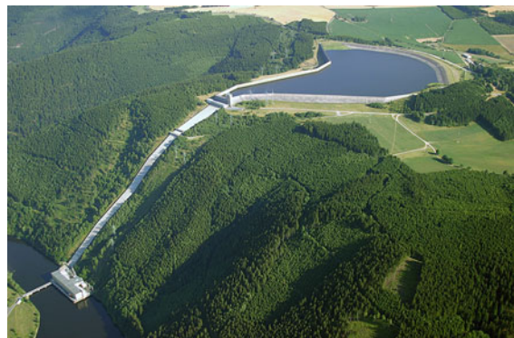
Fig. 26.83 Energy storage plant near Hohenwarte, Germany. The lake is filled with water if there is more power in the network than is needed. During times of shortage, the water is given back to the River Elbe, which can be seen at the bottom of the image (Photo: Vattenfall)
