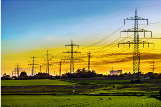
Fig. 26.65 Masts with 2 \times 3 380 kV power line phases in the upper part, and 2 \times 3 20 kV line phases in the lower part. At the top, a lightning conductor can be seen. (Photo: © okanakdeniz/stock.adobe.com)
