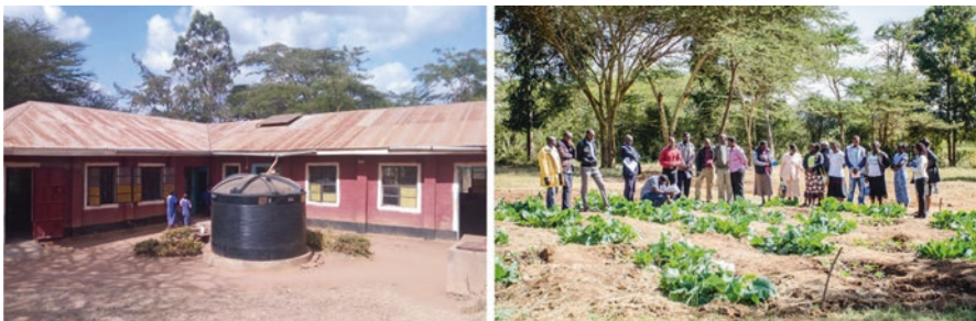
Fig. 14.1 Roof water harvesting system with solar and vegetable gardening projects at Watema Primary School
