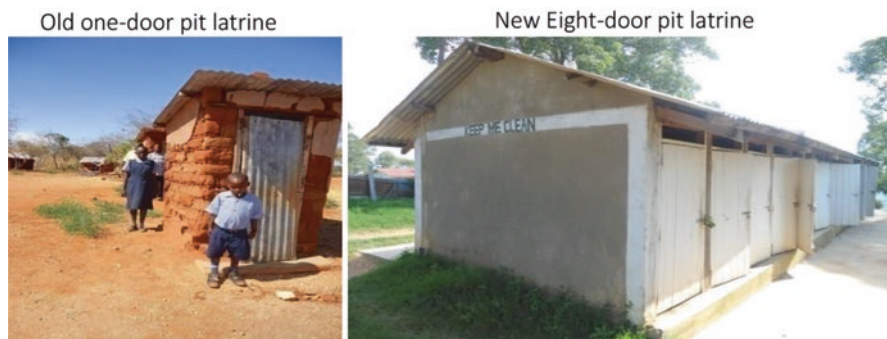
Fig. 14.2 Old and new latrines at Kirukuma Primary School. (Photos courtesy of Kirukuma Primary School-Kenya taken in August 2012)
