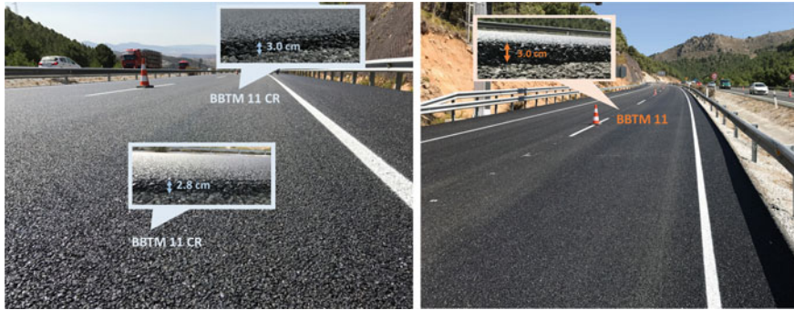
Fig. 4 Detail of the trial section before opening to traffic
