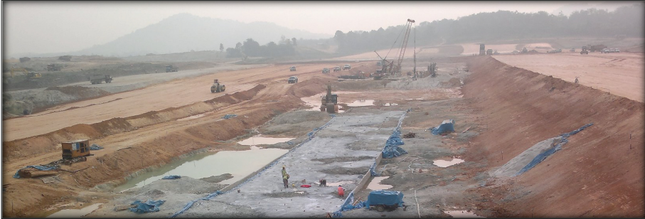
Fig. 4. Consolidation grouting on moderately weathered rock foundation
