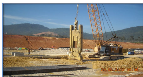
Fig. 3. Trenching for plastic concrete wall using clamshell bucket
