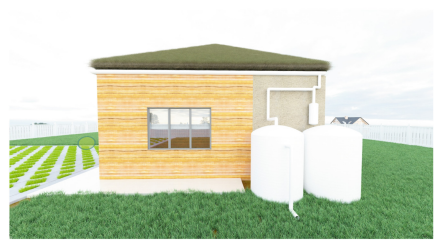
Rear view with rainwater harvesting tanks
