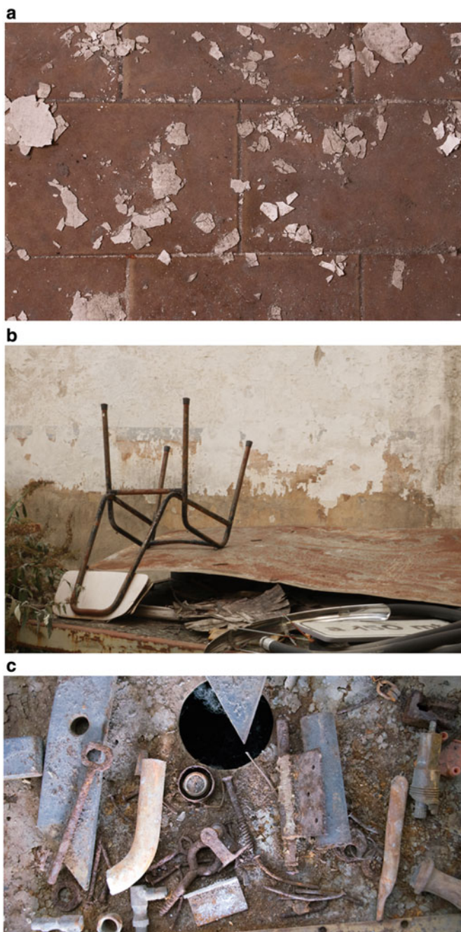
Fig. 2 Former warehouse of the State Railway, Varese (Italy), details; floor (a) furnitures (b) small objects (c). Photographs by Michela Albergati, Federica Borrello, Elena Grisa, Gennaro Merolla, Federico Nunziata, Giulia Turati
