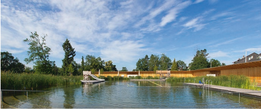
Fig. 13.6 Naturbad Riehen, built in the years 2010–2014 and located in Basel, Switzerland, the public pool designed by the architects Herzog and de Meuron, receives about 2000 bathers daily, cleaning does not depend on filters or chlorine, uses the vegetation that surrounds it, a process called phytodepuration. Photography: www.naturbadriehen.ch
