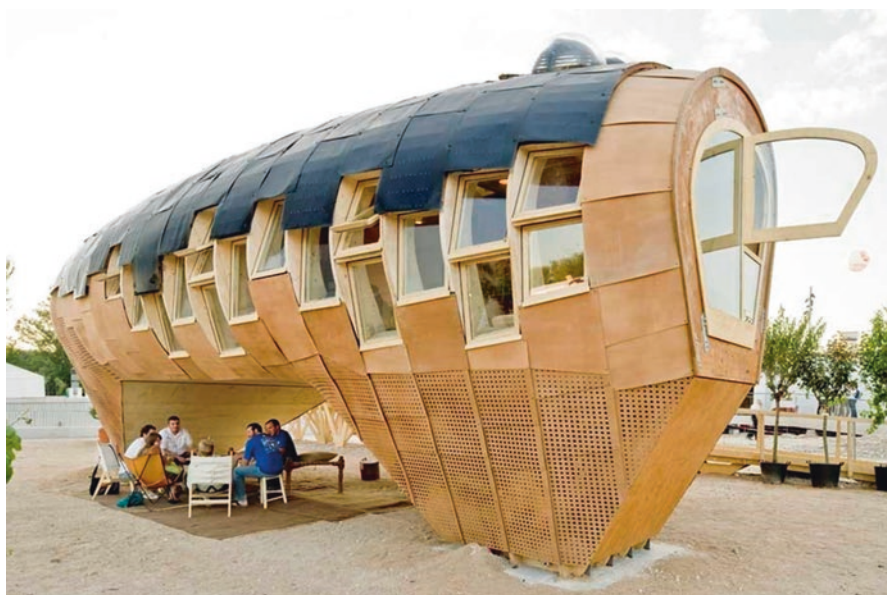
Fig. 13.5 Fab Lab House, designed in 2010 by the Advanced Architecture Institute of Catalonia (IAAC) in collaboration with MIT and the Fab Lab network. The house, by design, maximizes the collection of solar energy by having photovoltaic panels in its coverage depending on the movement of the sun. Photography: Fab Lab House
