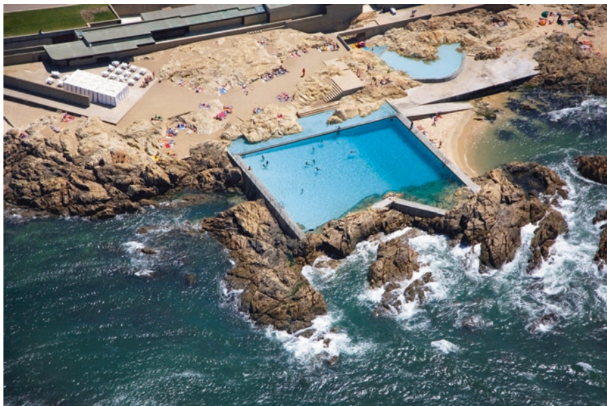
Fig. 13.2 Pools of Marés in Porto, Portugal, by architect Alvaro Siza (1966), takes advantage of the morphology of the beach to create pools with few materials and water from the sea itself. Its operation is subject to the rhythms of nature. Photography: Fernando Guerra and Sérgio Guerra
