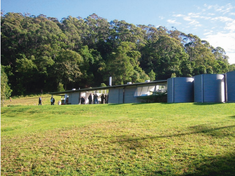
Fig. 13.3 Fletcher-Page House, by architect Glenn Murcutt (2000), among several other qualities about sustainability, the house also collects rainwater for later use. Photography: user Guess.Who / Flickr
