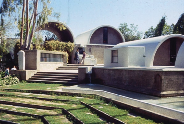
Fig. 13.10 Sanghat is the office of the architect Balkrishna Doshi (1981), in its design sustainability criteria were considered as the use of vaults that reflect solar radiation, the incorporation of vegetation for temperature control, the water path to humidify the facilities, among others. Photography: Nicholas Iyadurai
