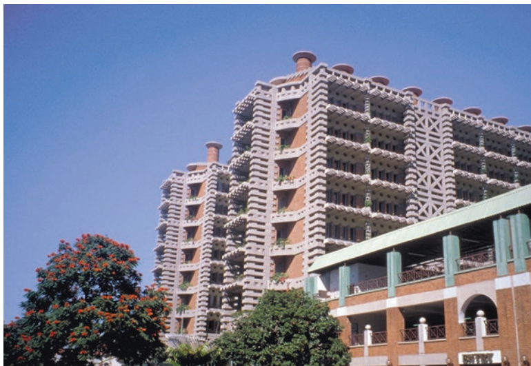
Fig. 13.4 Eastgate shopping center, in Harare, Zimbabwe. Designed by the architect Mick Pearce (1996), it uses the Venturi effect to provide fresh air during the day to the stores, the concept of thermal design was inspired by the structure of a termite mound. Photography: www.arup.com
