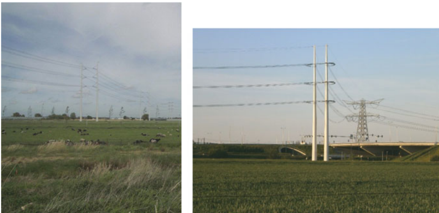
Picture 9 Wintrack towers in the Netherlands, here as a double-circuit 400 kV line with one system on each pole; left: suspension tower, right: tension tower ( Source Austrian Power Grid)
