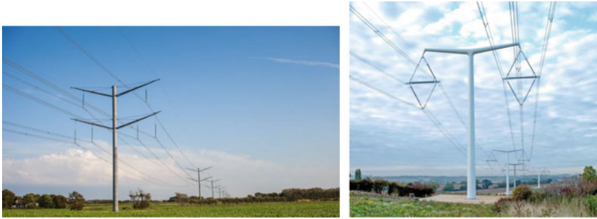
Picture 10 New 400kV tower design in Denmark (left) and in UK (right) (Source Bystrup architects)
