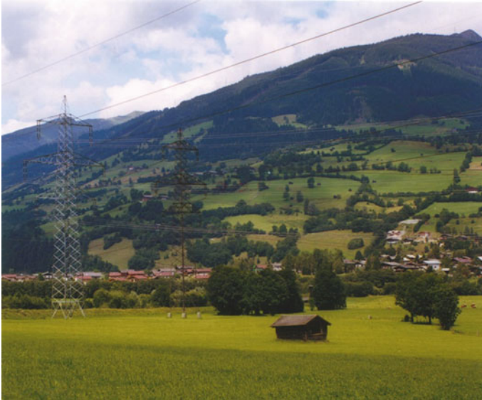
Picture 3 Two OHL towers with two systems 400 kV each can be seen. Left: galvanized steel tower, clearly visible; right “camouflage line” with dark green coated tower and conductors, nearly invisible [1]
