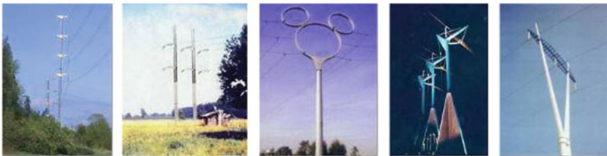
Picture 8 New tower design; from left: Finland, France, USA, Finland, Spain ( Source CIGRE publication 416)
