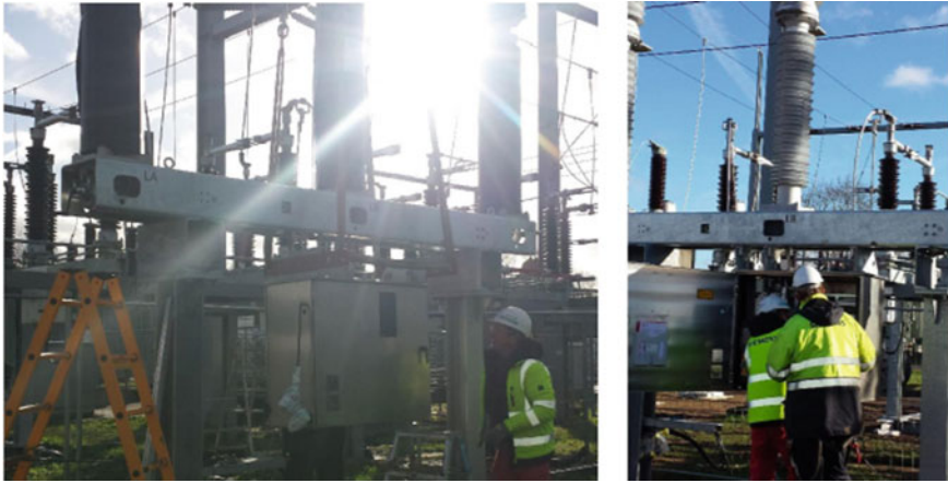
Fig. 9 Installation of Vacuum circuit breaker in 110 kV substation (courtesy of siemens)
