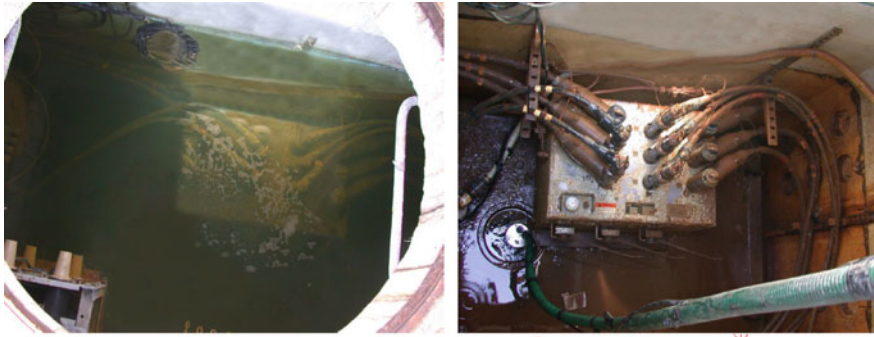
Fig. 20 27 kV, smart submersible SF 6 switch (courtesy of G&W electric co) [39]
