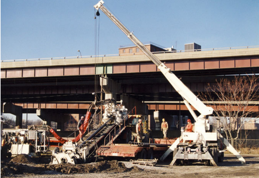
Fig. 2 A typical horizontal directional drilling rig
