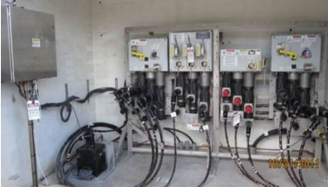
Fig. 19 38 kV, Smart, submersible Vacuum fault interrupter with reclosing capability
