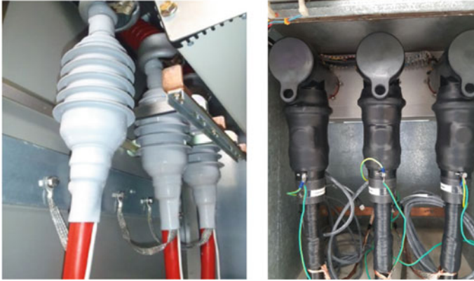
Fig. 41 Cable termination with combined LPIT embedded—on the left for air-insulated substation; on the right for gas-insulated substation
