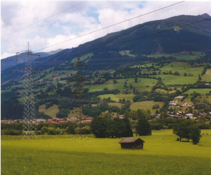
Picture 3 Two OHL towers with two systems 400 kV each can be seen. Left: galvanized steel tower, clearly visible; right “camouflage line” with dark green coated tower and conductors, nearly invisible [1]
