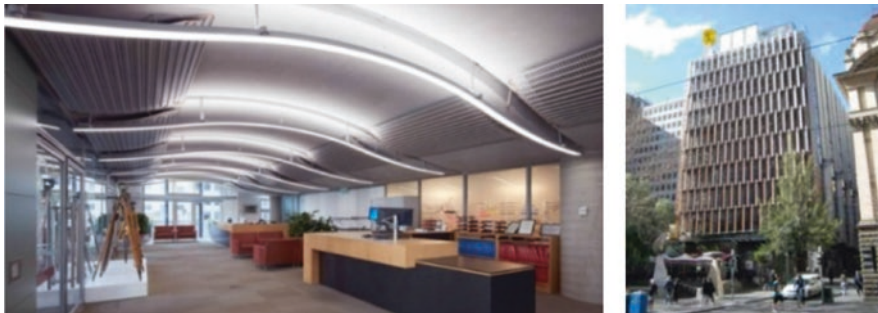
Fig. 11 Interior and exterior of the CH2 building, Melbourne, Australia. Image source: https://www.researchgate.net/publication/262857243_Biomimetic_design_for_climate_change_adaptation_and_mitigation
