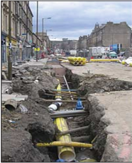
Works are causing disruption to drivers [7]
