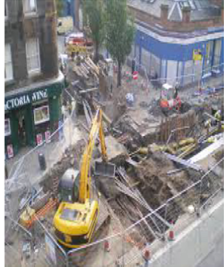
Utility diversion works delayed construction [8]
