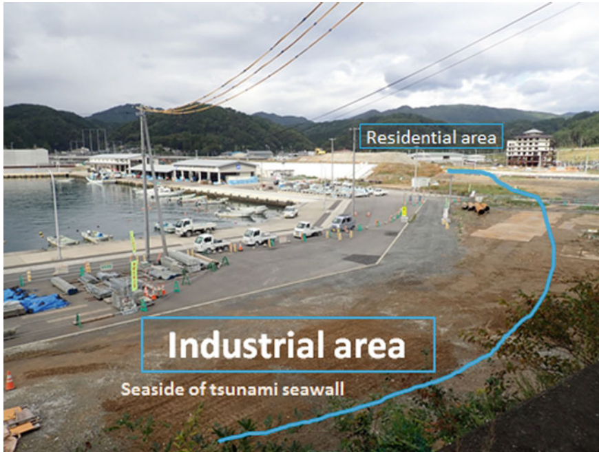
Fig. 5 Taro area in Miyako City, where a 14.7 m high tsunami breakwater has been constructed. Work activities will be carried out on the seaward side of the seawall during the day, and workers will return to the landward side of the seawall at night
