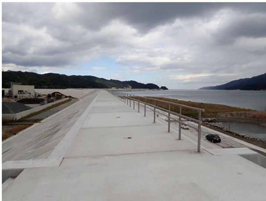
Fig. 4 A huge seawall constructed in Miyako, Iwate Prefecture. The tidal land area was infilled to a width of 10–30 m
