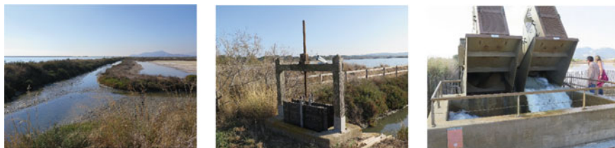
Fig. 6 Salins des PESQUIERS salt marshes (eastern Provence, France). Left: general view, with a canal. Centre: a lock. Right: the pump that lowers the water level in the pans and discharges the water into the belt canal, and from there into the sea. Photographs © Charles F. Boudouresque
