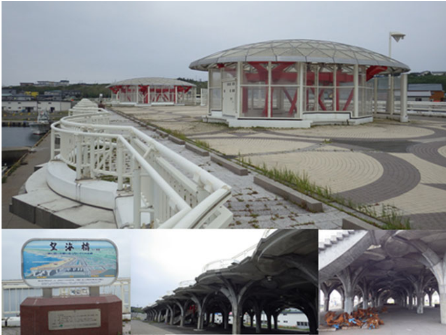
Fig. 6 Bokai Bridge built for tsunami emergency evacuation in Okushiri Island after the earthquake and tsunamis in 1993
