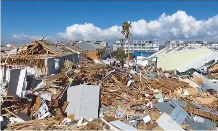
Fig. 8.2 Hurricane Michael damage. (Courtesy of Wikimedia Commons)
