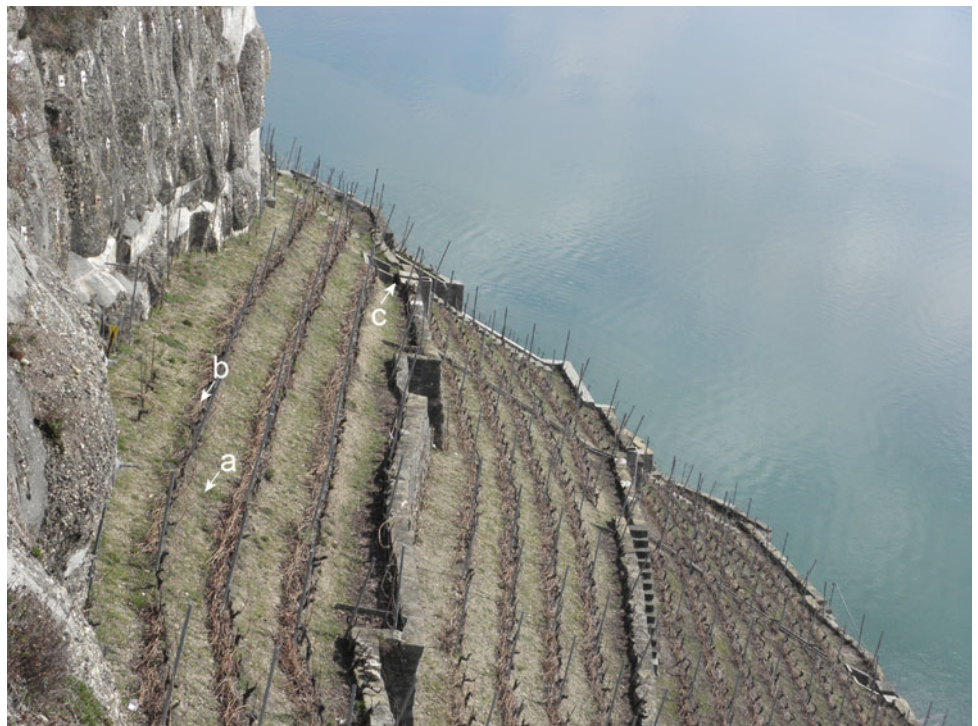
Fig. 8.10 Techniques for mitigating soil erosion. a grass soil cover; b dead branches left on the soil; c system for water collection (photo E. Reynard)
