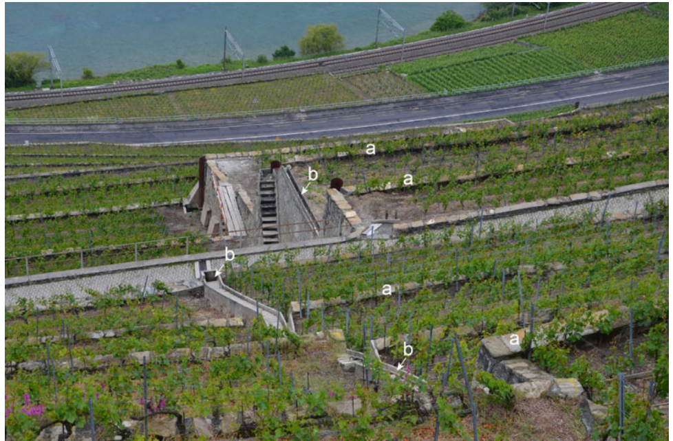
Fig. 8.9 Hydrological and sediment flux management. a Upper elevated part of the wall; b artificial channels collecting water (photo E. Reynard)
