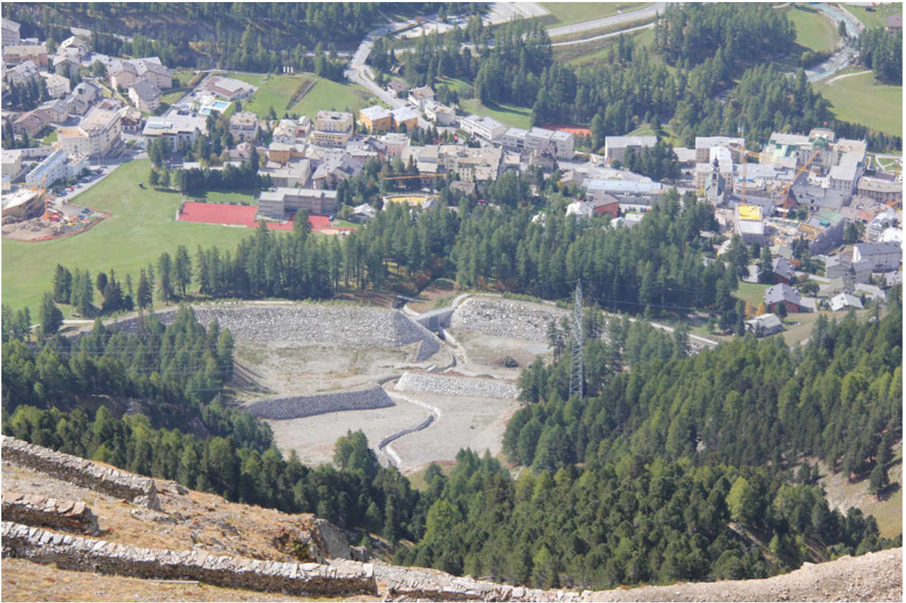
Fig. 28.8 Avalanche—and debris flow retention dam above Pontresina (photo M. Heggli)
