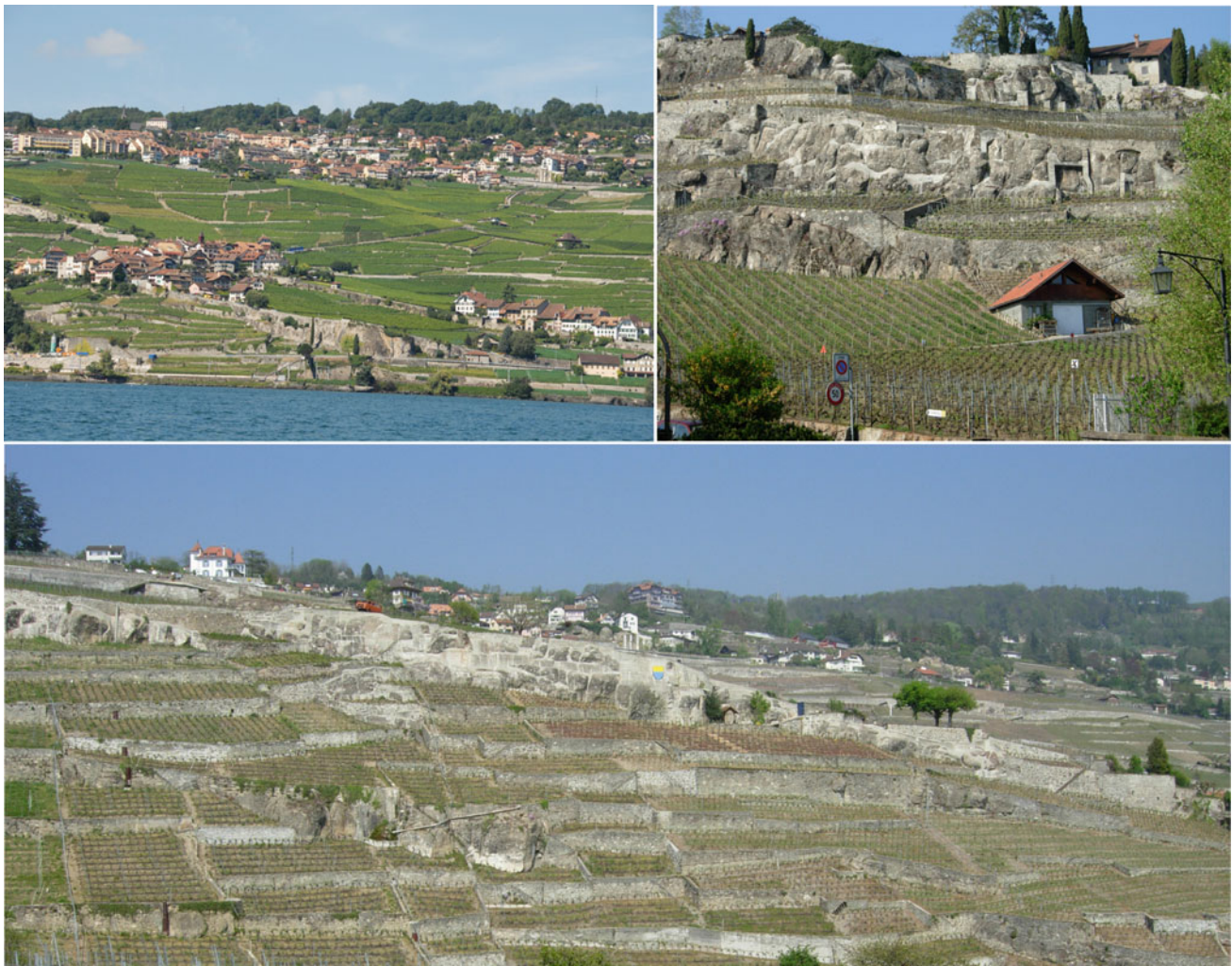
Fig. 8.8 Conglomerates banks structuring the vineyard slopes and maintenance works (photos E. Reynard)
