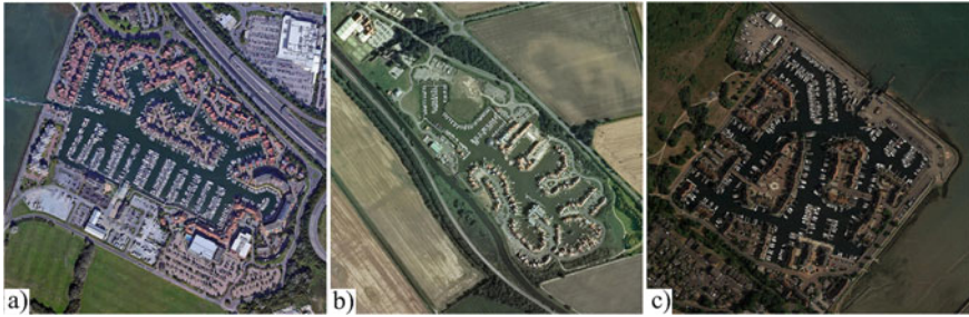
Fig. 1 Architectural–planning imitation of a small settlement structure: a Port Solent, Portsmouth, UK; b Burton Waters (marina village), Lincoln, UK; c Hythe Marina Village, Southampton, UK [8]
