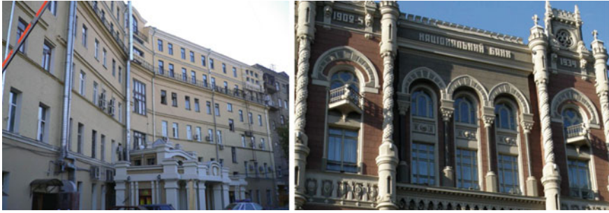
Fig. 1 Reconstruction of the buildings with additional storey erection
