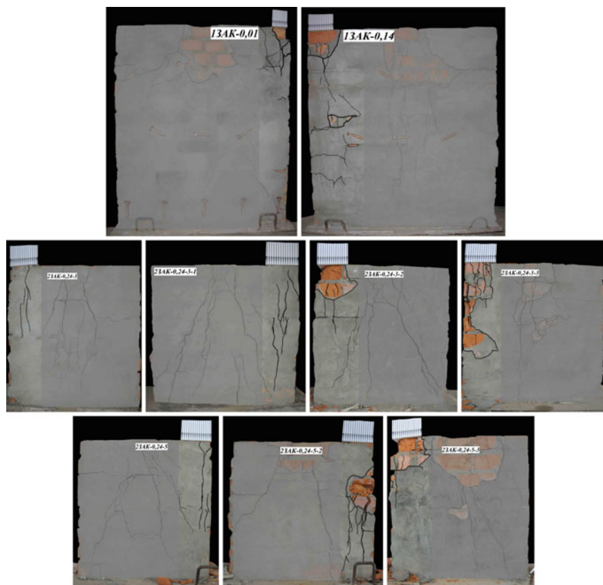
Fig. 7 Nature of the reinforced masonry specimens destruction under edge local compression
