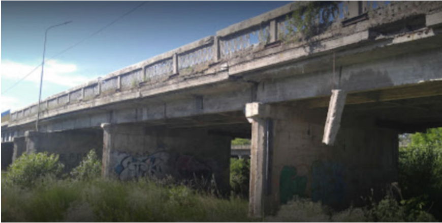
Fig. 4 View of the bridge structure across the Borova River, Luhansk Oblast
