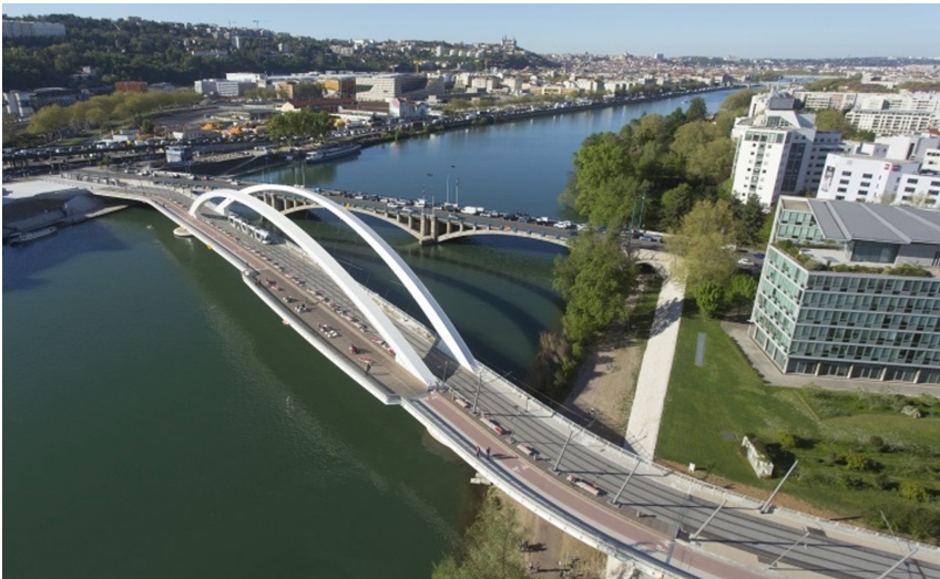
Fig. 2. Raymond Barre bridge (source: Bouygues construction)
