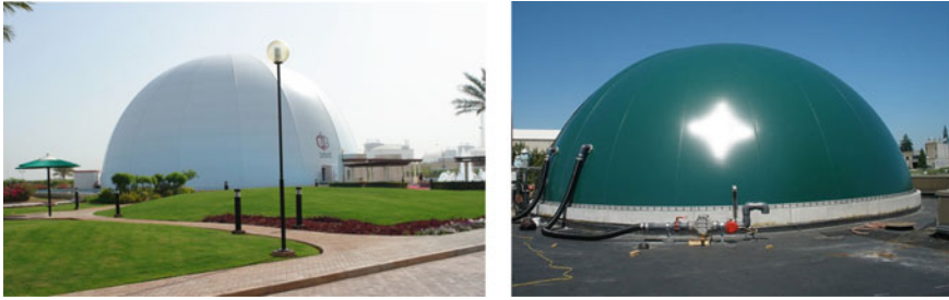
Fig. 61.1 Thin-walled air-inflated structures of hemispherical shape: Roofing from Architen Landrell in Qatar (left), Gasholders of the company Sattler Ceno TOP-TEX GmbH (right)
