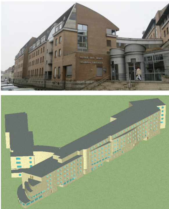
Fig. 2.7 Top: Lavoisier student residence in Douai. Bottom: Lavoisier student residence in 3D
