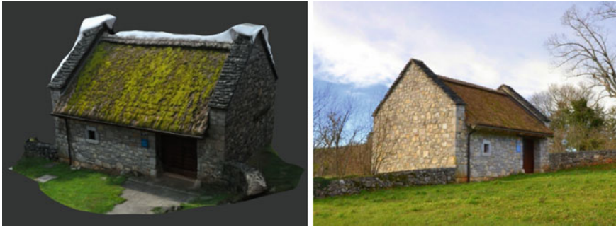
Fig. 1.5 Left: a 3D model of a real thatched barn created with stereophotogrammetry. Right: the barn used to create a 3D model
