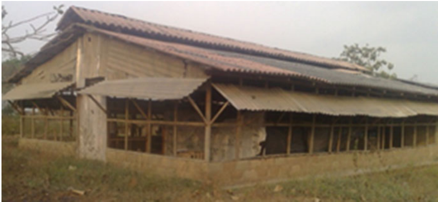
Fig. 3 Low-walled broiler housing units
