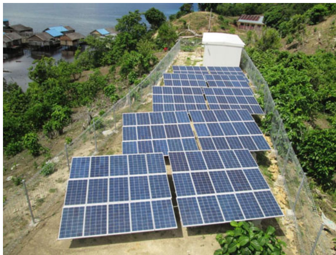
Fig. 1 Indonesian government has been massively deploying over 700 PV mini-grids from 2012 to 2018 with installed capacity ranging from 10 to 150 kWp. Some of these sites can be viewed here: http://remap-indonesia.org/ . Photo GIZ
