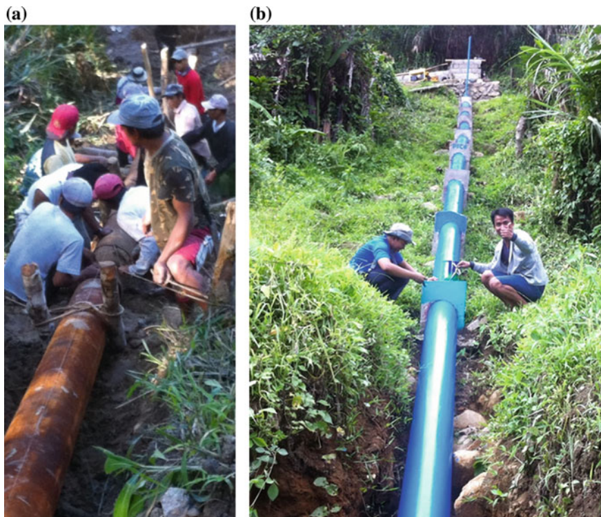
Fig. 20 a Hauling of the steel material and b completed penstock
