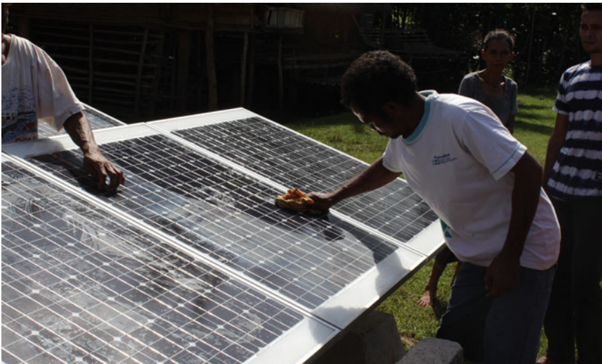
Fig. 9.6 Demonstration by a village representative on how to maintain the solar PV system
