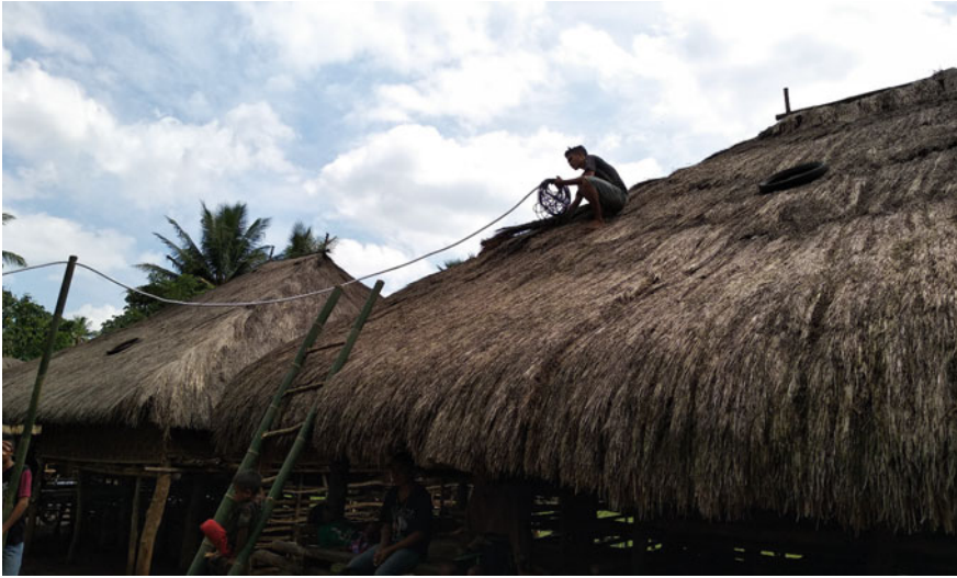
Fig. 9.5 Villager pulling a cable to allow the house to receive electricity
