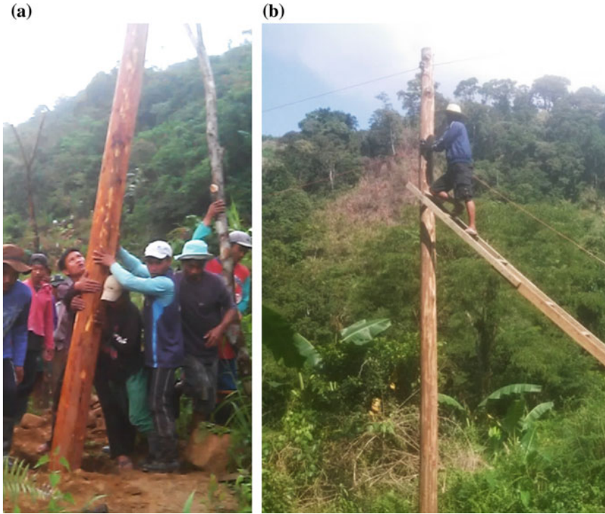
Fig. 27 a Installation of electrical post and b wiring
