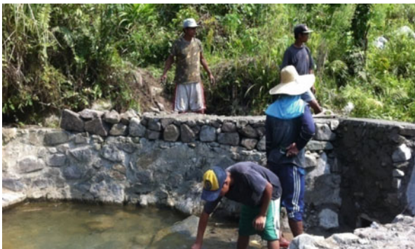
Fig. 14 Intake and weir using stone masonry
