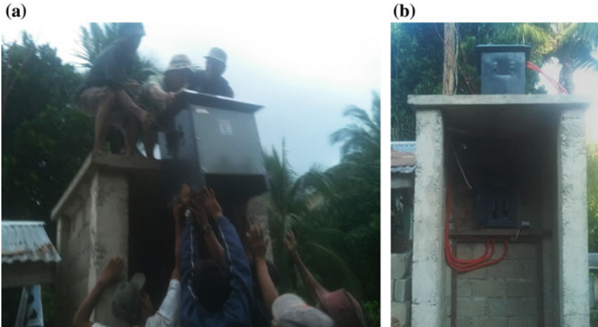
Fig. 26 a Installation of transformer and b completed substation
