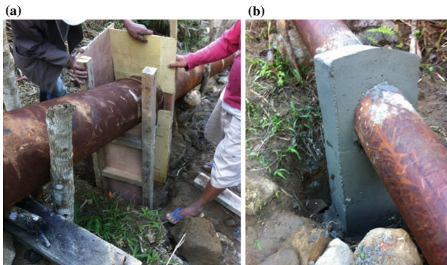
Fig. 21 a Anchor block wooden forms and b completed anchor block
