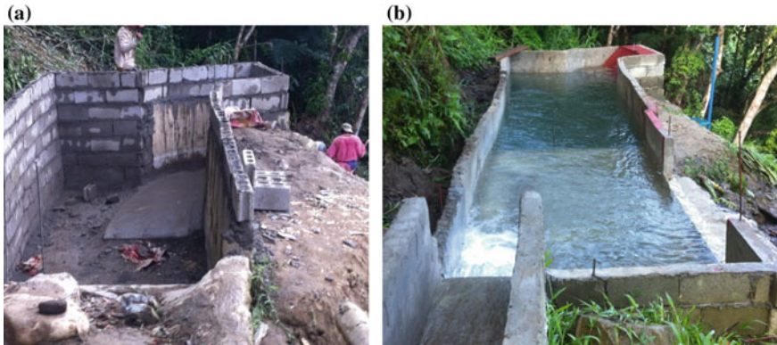
Fig. 19 a Concrete hollow block forebay during construction and b completed forebay
