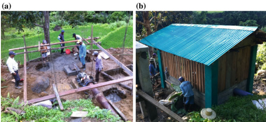
Fig. 24 a Setting the powerhouse foundation and post and b completed powerhouse
