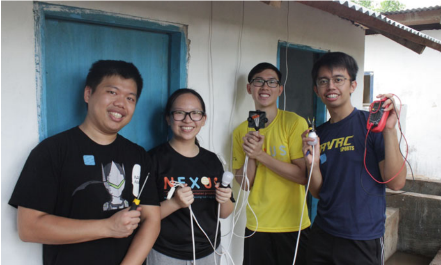
Fig. 9.12 MKP team installing the light bulbs and electrical box
