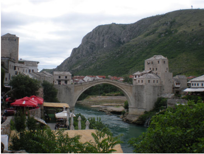
Fig. 11.1 Stari Most, the old bridge in Mostar spanning the Neretva River (photograph by Nicholas Wise)
