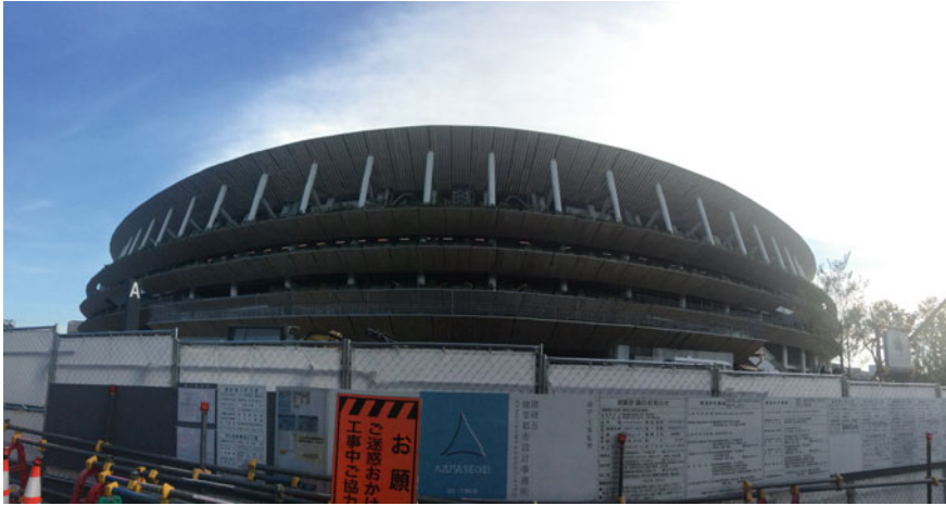
Fig. 10.3 Olympic Stadium (photograph by Takamitsu Jimura)
