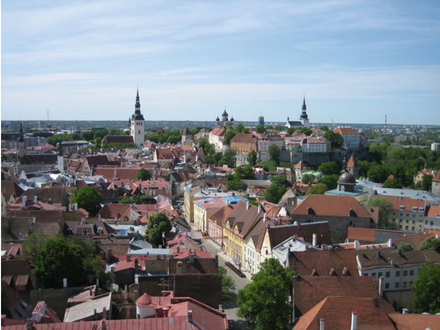
Fig. 5.1 A view from the St. Olav's Church tower's observation platform to the Old Town of Tallinn, a UNESCO World Heritage Site, which morphologically consists of Lower and Upper Towns, in 2006 (photograph by Aleksandr Michelson)
