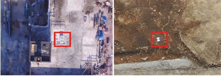
Fig. 5.4 Example of GCPs (marked in red) place on the construction site for registering the Reality models to BIM or real-world coordinate system
