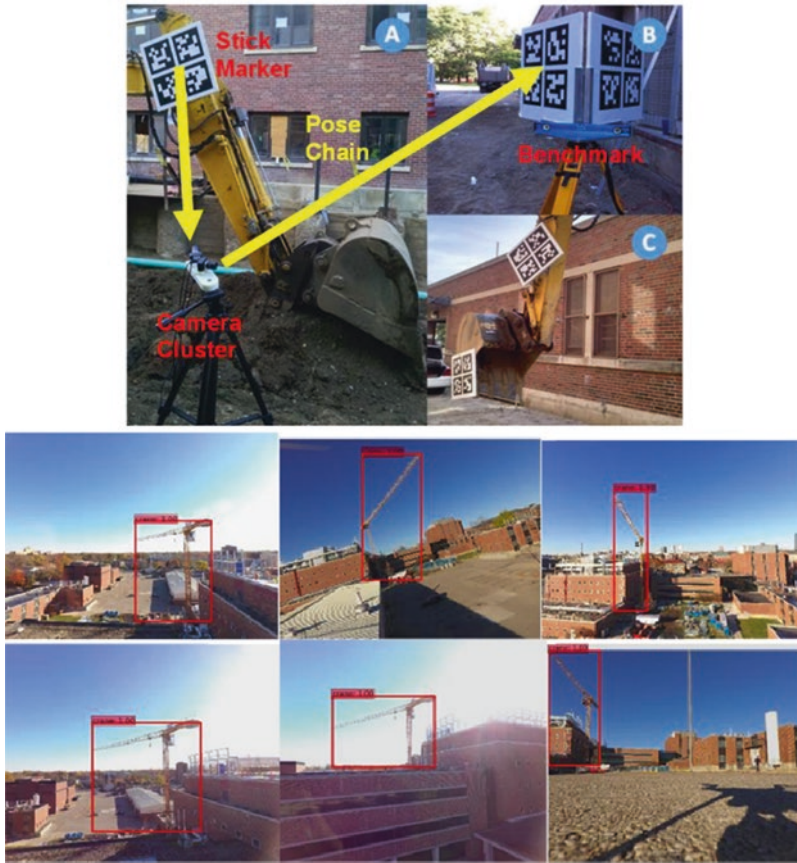
Fig. 10.3 Computer vision techniques for equipment pose estimation: marker-based (Yang et al. 2013) and machine-learning based methods (Roberts et al. 2017)
