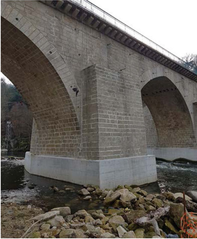
Fig. 2 Concrete belts at pillars P2 and P3
