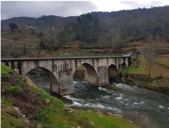
Fig. 1 Bridge of Cavez before the rehabilitation (March 2018)
