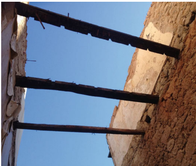
Fig. 2 Containment of facades with two existing beams
