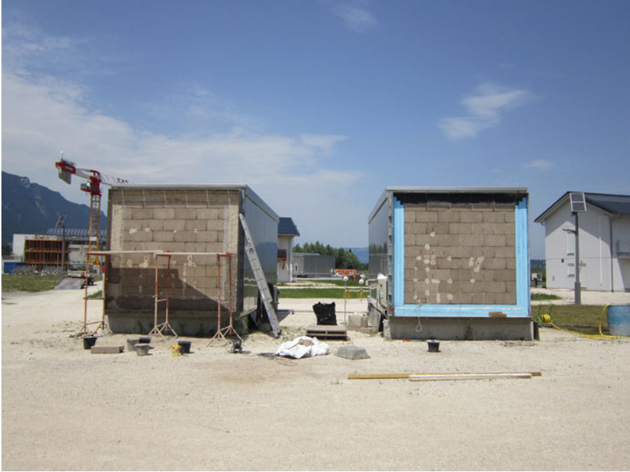
Fig. 6.12 Experimental setup of the two PASSYS test cells at Le Bourget du Lac, France (Bejat et al. 2015) © CEA
