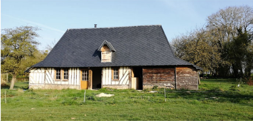
Fig. 2.7 A half-timbered building in Normandie, France, dating from the early nineteenth century. The walls and slabs were renovated using different solutions based on hemp concrete. (Source: with the kind courtesy of Florence Collet (Rennes, France) and Yacine Ait Oumeziane (Belfort, France))
