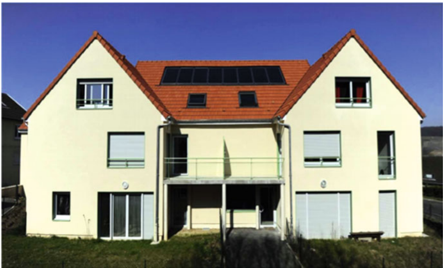
Fig. 6.14 View of the southern façade of the building located at Fleury la Riviere, France; (Costantine et al. 2018) © Foyer Rémois
