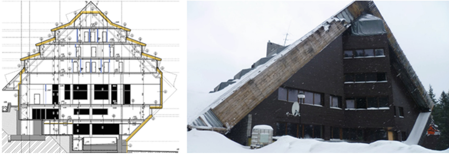
Fig. 2. Cross section of the building and view after fire.
