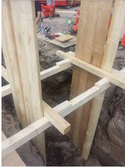
Fig. 2. Provisional sheeting (Author)
