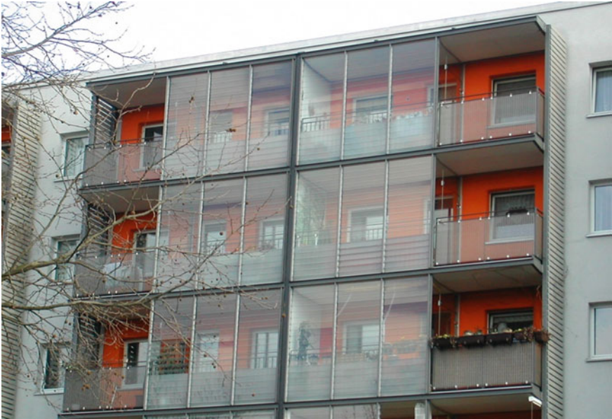
Fig. 9.2 Energetically renovated facade of an old social housing building in Dresden (D). Credits The Author 2012
