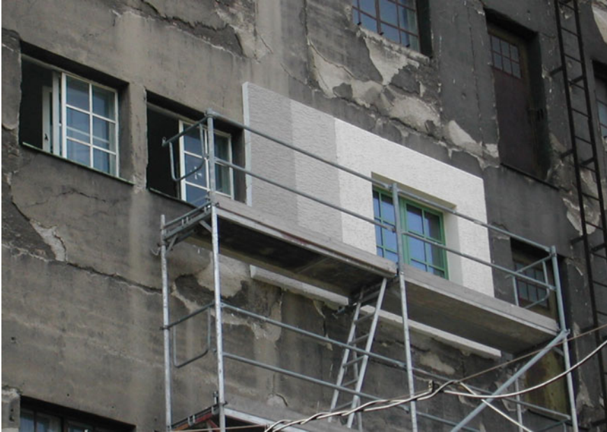
Fig. 9.1 New façade sampling for an energy retrofit project in Dresden (D). Credits The Author 2012
