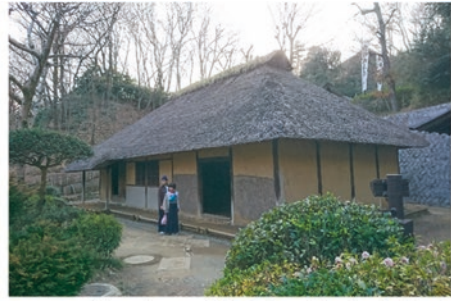
Japanese village house with adobe walls, thatched roof and “engawa” (porch) Yamanashi Prefecture – XVII-th Century, Village Museum, Tokyo Photo: Ana-Maria Dabija
