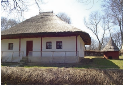
Romanian village house with adobe walls, thatched roof and “prispa” (porch) Dobrogea – XVIII-th Century, Village Museum, Bucharest, Romania Photo: Ana-Maria Dabija
