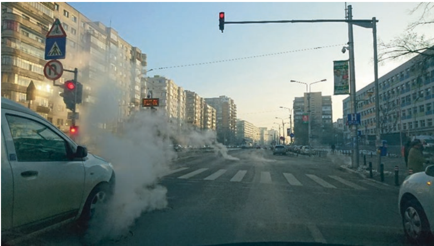
Fig. 15.5 A winter morning in Bucharest, 2019. The heat – hot steam – is lost in the ducts that lead from the thermoelectric power stations to the buildings. (Photo: Ana-Maria Dabija)
