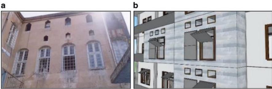
Fig. 14.5 (a) “Bird windows” in a traditional Gaziantep house, (b) contemporary interpretation of “bird windows” in the design
