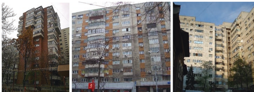
Fig. 15.6 Buildings of the 1980s: facing the boulevard and facing the inner courtyard/second line of buildings. (Photo Ana-Maria Dabija)
