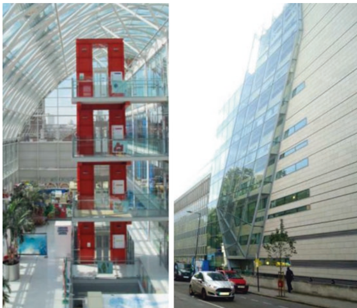
Fig. 10.4 On the left, the curved glass roof of Evelina London Children’s Hospital that due to the absence of mechanical air conditioning system and the high temperature during in the summer of 2006, the whole hospital building was overheated, putting patients in danger. On the right, the glass building volume of Great Ormond Street Hospital in London helps in the ventilation of the hospital and simultaneously reduces energy consumption. (Photos: A. Kyrkou)
