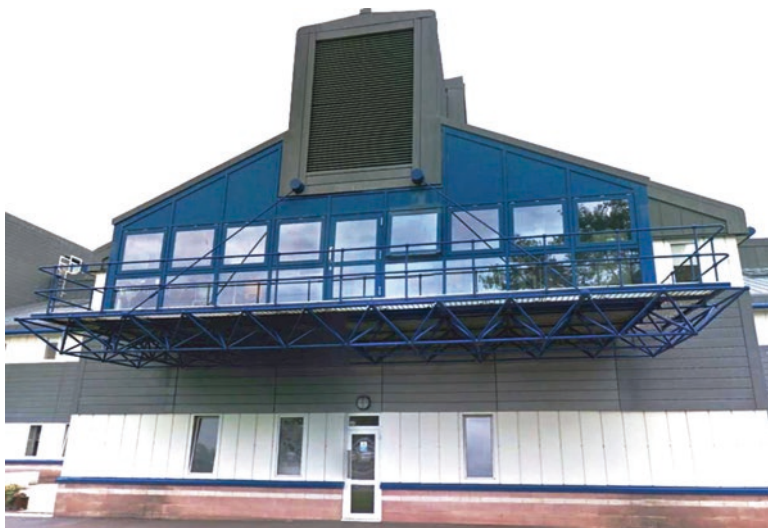
Fig. 10.3 At St. Mary's Hospital (1991), ABK architects, Isle of White, UK, the sustainable approach (low energy) played also a fundamental role on the facades of the building and the overall exterior appearance of the hospital. (Photo: A. Kyrkou)
