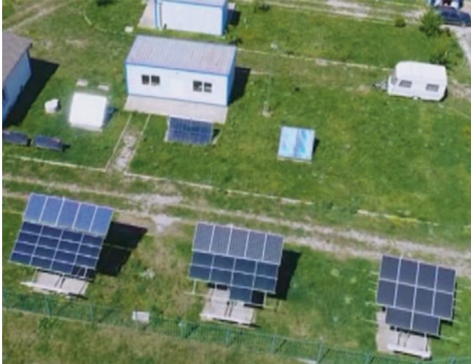
Fig. 2.11 Experimental platform at the Technical University of Sofia with five PV systems from five technologies, mounted on three solar trackers
