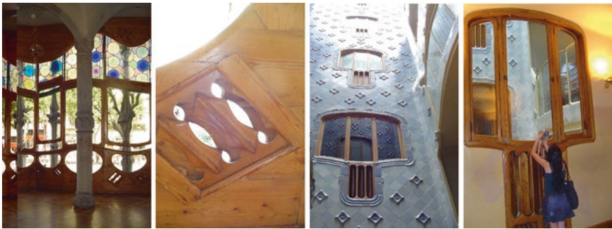
Fig. 6.5 Antonio Gaudí – cross-ventilation in Casa Batlló, designed in 1904. The house is provided with windows and parapets that allow opening and closing of the acir being evacuated in the central “well”, in fact an inner courtyard. (Photos: Ana-Maria Dabija)
