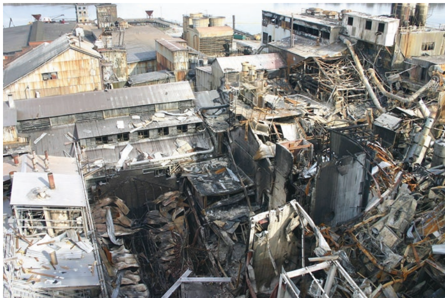
Fig. 1.7 Aftermath of a sugar dust explosion at a sugar refinery, 2008. (Source: Chemical Safety Board, Wikipedia)
