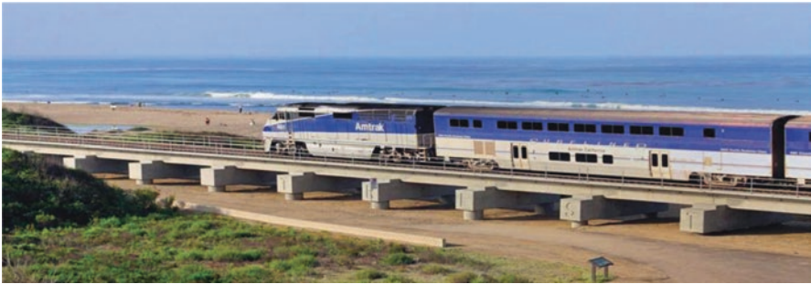
Fig. 14 Los Angeles to San Diego (LOSSAN) rail corridor that follows the sea coast and crosses low-lying areas on trestles [26]
