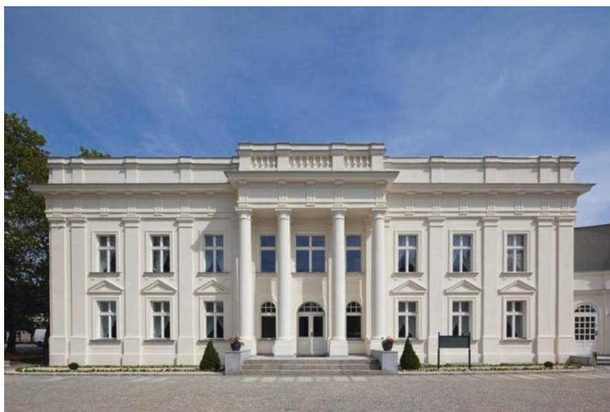
Fig. 2 A part of Turzno Palace after restoration. (With the permission of the copyright holder R. Predenkiewicz)
