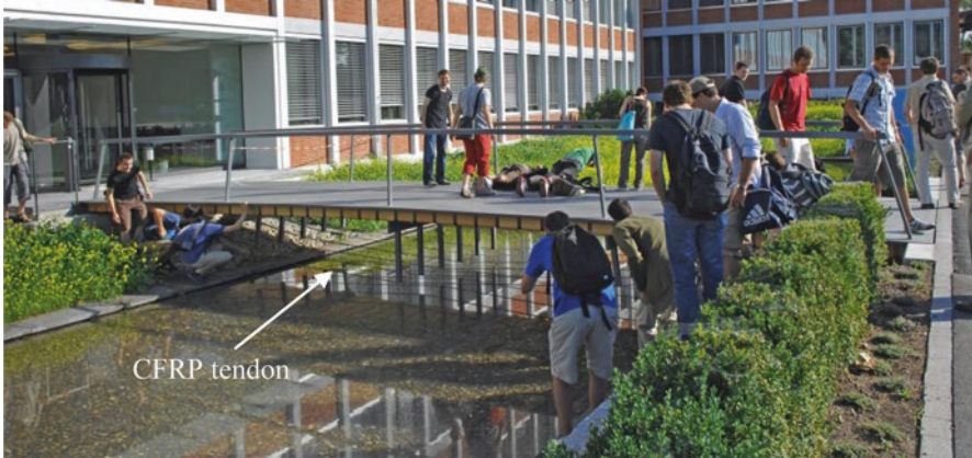
Fig. 20 Bowstring arch bridge fully supported by filigree but very powerful CFRP tendons
