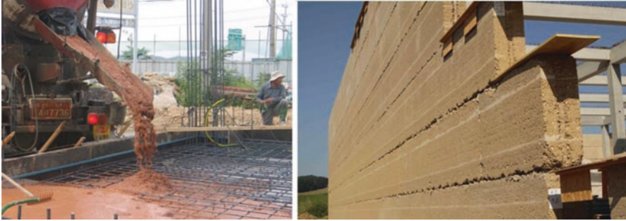
Fig. 13 Concrete technologies applied to construction with raw earth. Left: slab fabrication with ready-mixed pourable earth formulated with only ~10% water and clay dispersants (University of Mokpo, South Korea). Right: assembling pre-fabricated rammed earth elements during construction of the Ricola Herb Center, Switzerland (Jacques Herzog and Pierre de Meuron Architects; Engineering: Lehm Ton Erde GmbH)
