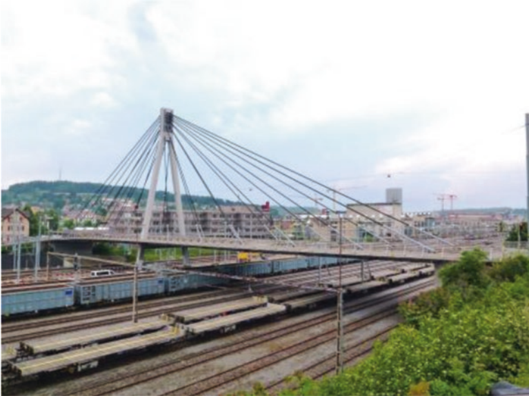
Fig. 6 Stork Bridge, Winterthur, with two CFRP stay cables installed in 1996. Load-carrying capacity of each cable: 12 MN
