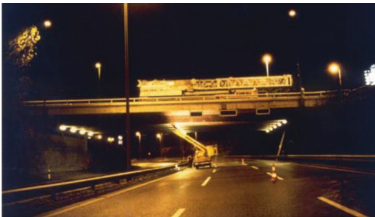
Fig. 4 Loading test on Ibach Bridge after strengthening with CFRP laminates
