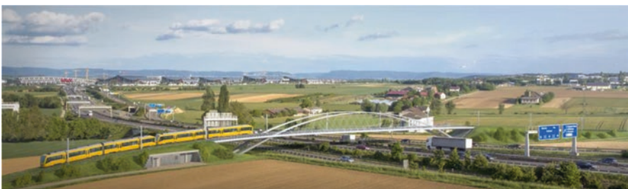
Fig. 21 Network arch bridge designed by Schlaich Bergermann Partner for the city public transport operator Stuttgarter Straßenbahnen (SSB) fully suspended on CFRP hangers. Source of rendering: Stuttgarter Straßenbahnen AG
