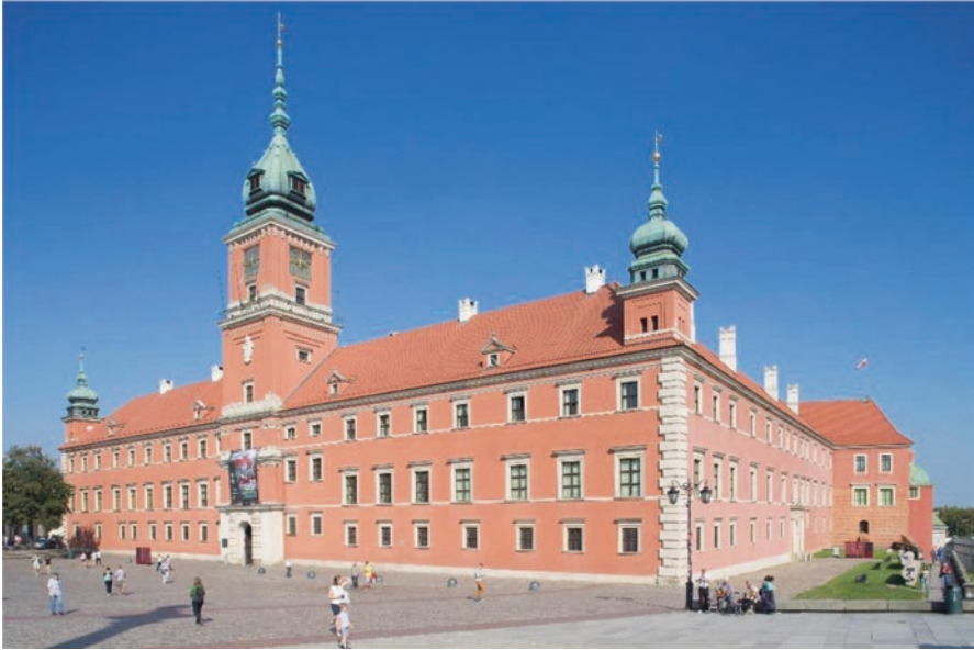
Fig. 6 The Royal Castle in Warsaw (Poland): the state after renovation (2017). (Author P. Ostrowski. With the permission of the copyright holder Narodowy Instytut Dziedzictwa (National Heritage Board Poland))
