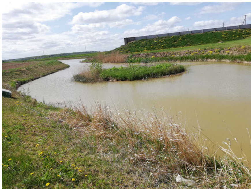
Fig. 6 Surface flow constructed wetland in farm Mezaciruli. Author Linda Grinberga
