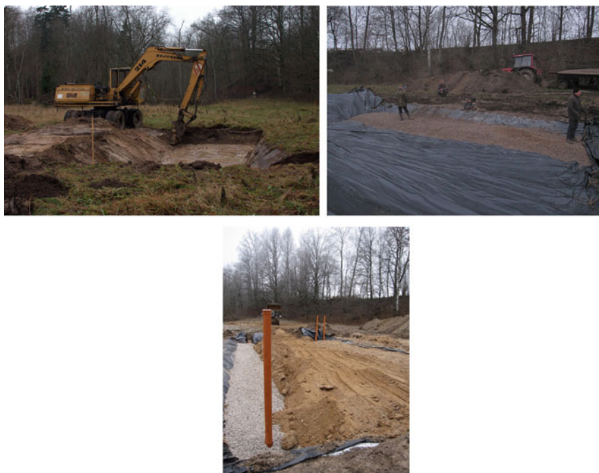
Fig. 5 The building process of the constructed wetland in Valti. Author Vanda Valtenberga
