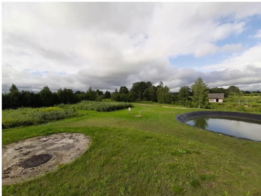
Fig. 4 Two vertical subsurface flow constructed wetlands in Tinuzi. Author Ugis Plaudis
