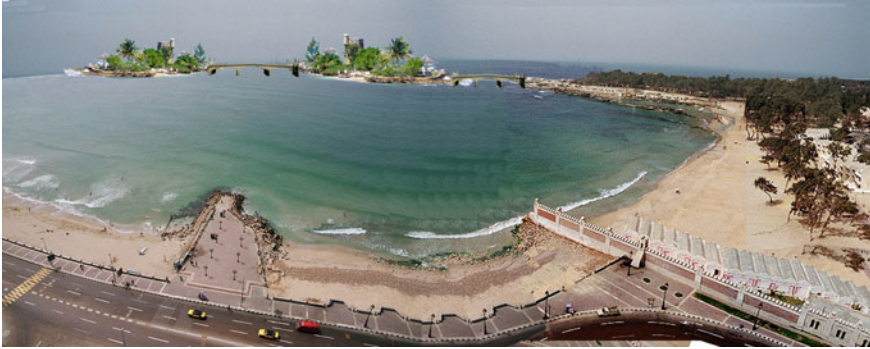
Fig. 14.31 A living shoreline for the coastal area of Alexandria. It illustrates protection of beaches against Tsunamis and severe storms
