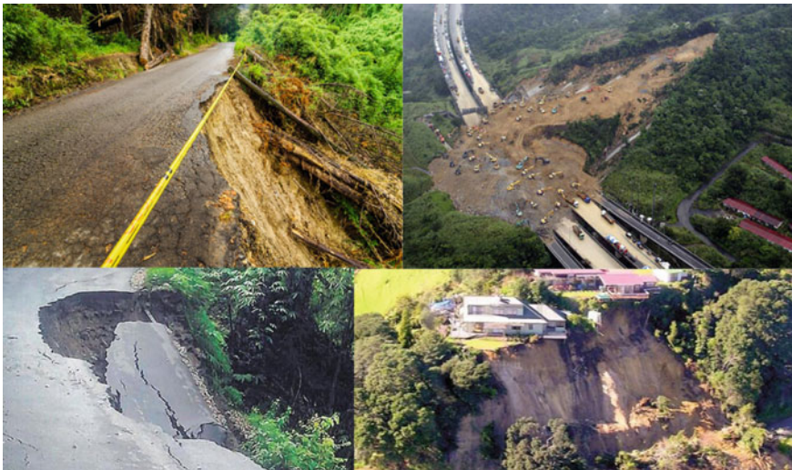
Fig. 6.3 Landslides on the slopes and inclines (Protić and Bonić 2018)
