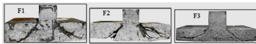
Fig. 6.9 Saw-cut of the failed footings (Bonić et al. 2017)
