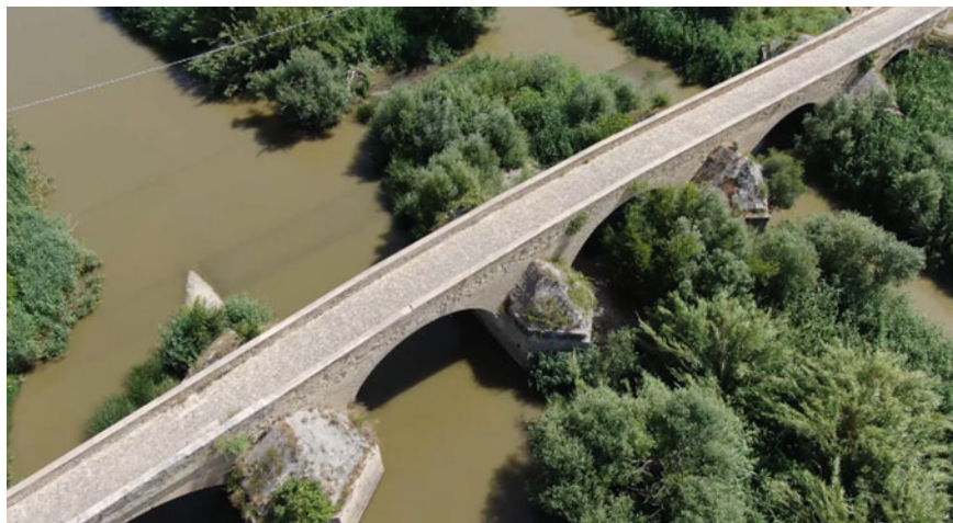
Fig. 5 Aerial view from the drone of the bridge
