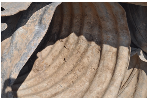
Fig. 17.4 Each of those ducts provide the desired amount of air to the bulk potatoes piled above the ducts
