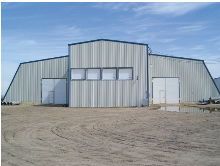
Fig. 17.2 All facilities need a strong foundation, insulation, protection from the elements, climate controls, ventilation system, and temperature controls to provide a suitable environment for potatoes. Modern storage facilities integrate air and humidification systems that allow year-round storage with minimal loss
