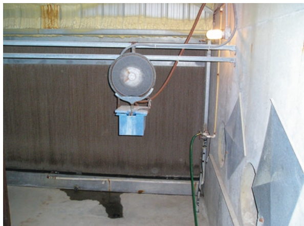
Fig. 17.14 Examples of humidification equipment in storages: evaporative cooling pad and centrifugal humidifier
