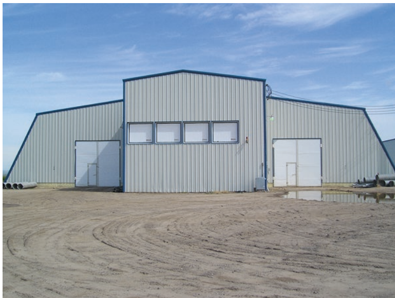
Fig. 17.2 All facilities need a strong foundation, insulation, protection from the elements, climate controls, ventilation system, and temperature controls to provide a suitable environment for potatoes. Modern storage facilities integrate air and humidification systems that allow year-round storage with minimal loss
