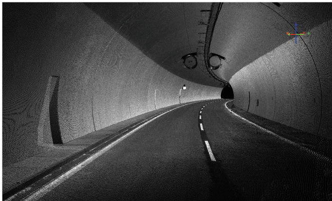
Fig. 1. Point cloud from experimental measurement of highway tunnel - Považský Chlmec 27. September 2017
