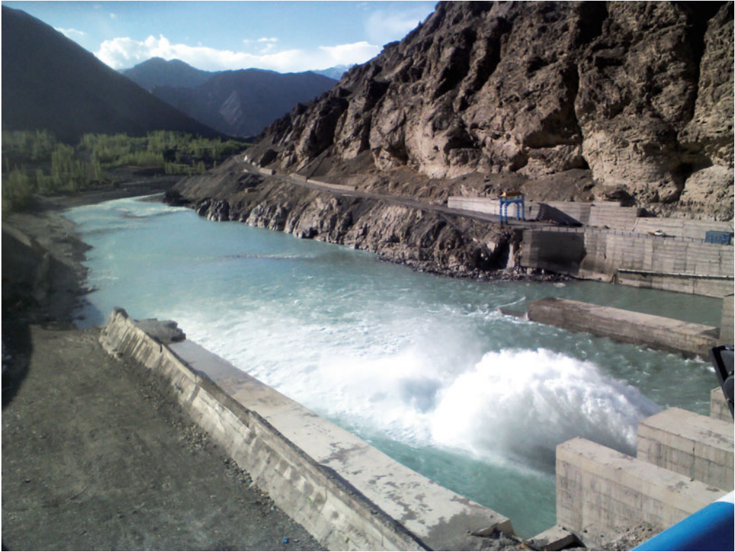
Fig. 7.10 Nimoo Bazgo Power Project, situated at Alchi village, on the Indus River in Ladakh. Credit Mehrajmir13 (CC BY SA 4.0, https://creativecommons.org/licenses/by-sa/2.0/ )
