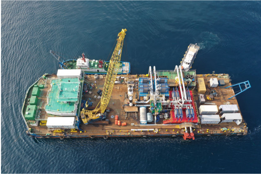
Fig. 14.13 1 MW Ocean Thermal Energy Conversion plant field experiment in Korea waters (© Hyeon-Ju Kim, Korea Research Institute of Ships and Ocean Engineering)
