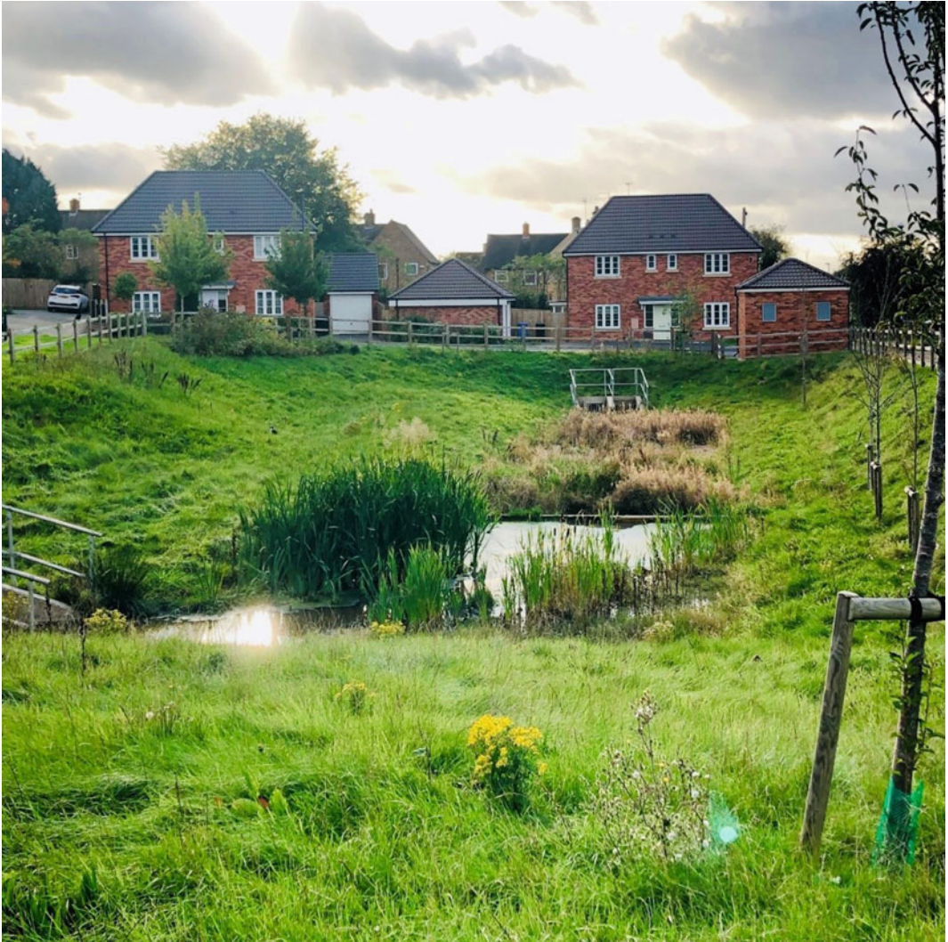
Fig. 11.6 Example of a retention sustainable drainage system installed in a new housing development in Derby, UK. Photo by author © UKRI (used with permission)
