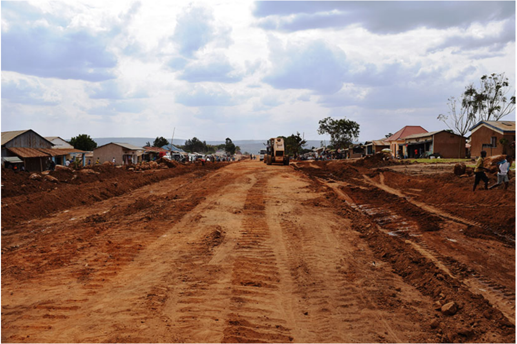
Fig. 9.1 Road construction in Tanzania. Credit Joel C. Gill
