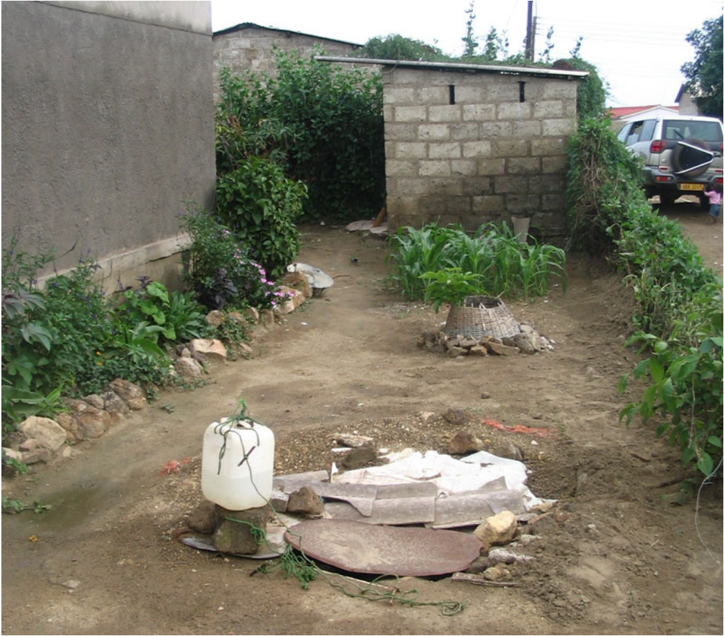
Fig. 6.12 Close proximity of groundwater well and pit latrine in peri-urban area of Lusaka, Zambia. Credit Kenedy Mayumbelo (reproduced under a CC BY 2.0 license, https://creativecommons.org/licenses/by/2.0/ )
