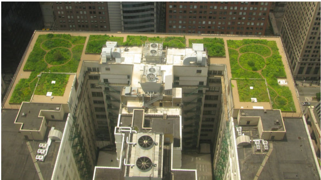
Fig. 11.9 Green roof on Chicago City Hall. This approach can improve insulation, provide habitats for biodiversity, and lower urban air temperatures. Adapted
