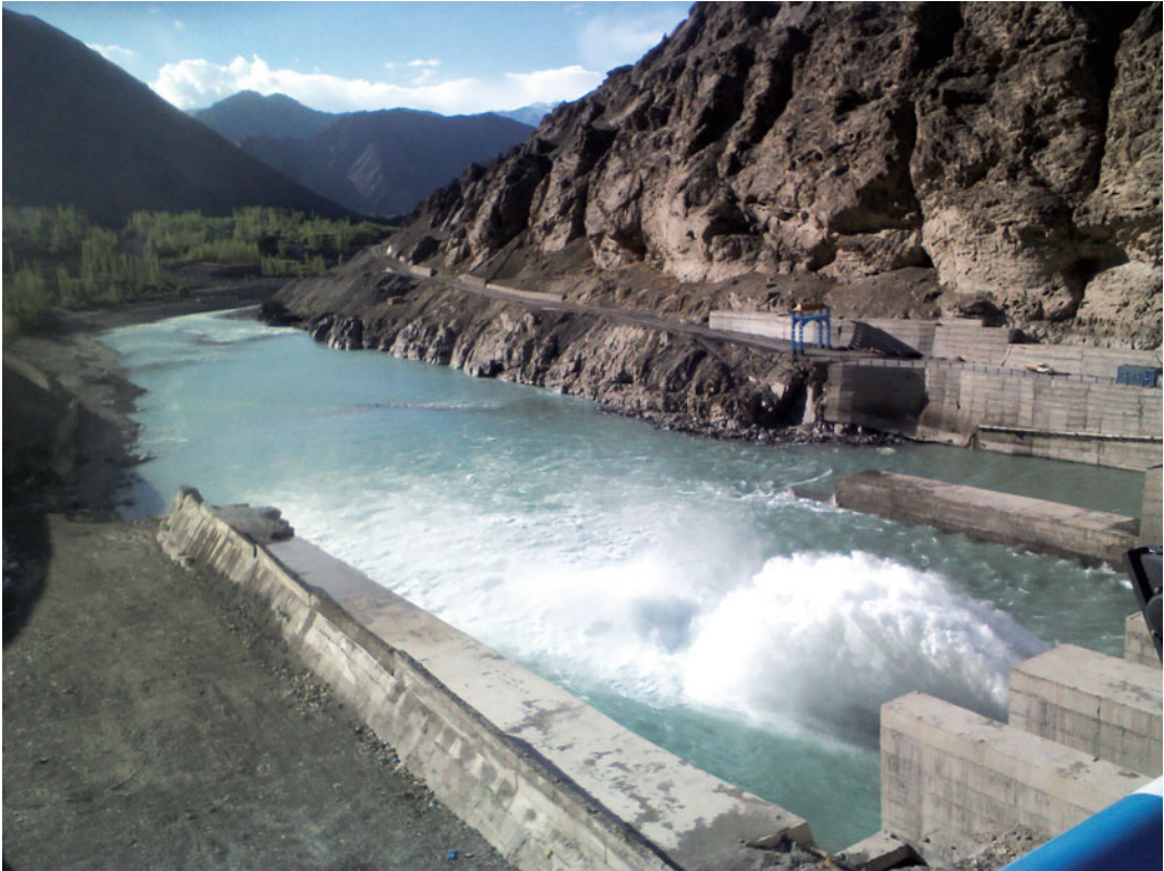
Fig. 7.10 Nimoo Bazgo Power Project, situated at Alchi village, on the Indus River in Ladakh. Credit Mehrajmir13 (CC BY SA 4.0, https://creativecommons.org/licenses/by-sa/2.0/ )
