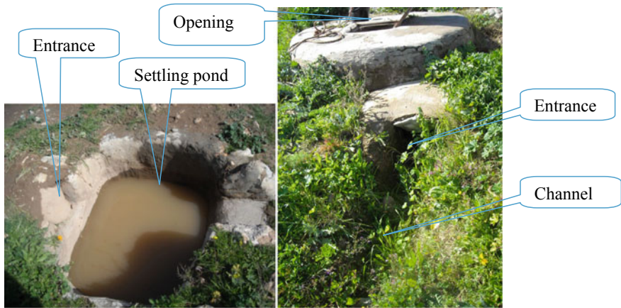
Photo-13.1 Detail of a traditional reservoir (matfia) and its compones
