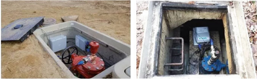
Fig. 12.9 Monitoring water mains through smart acoustic correlators linked to GIS. Courtesy Echologics and Mueller Co. [19]
