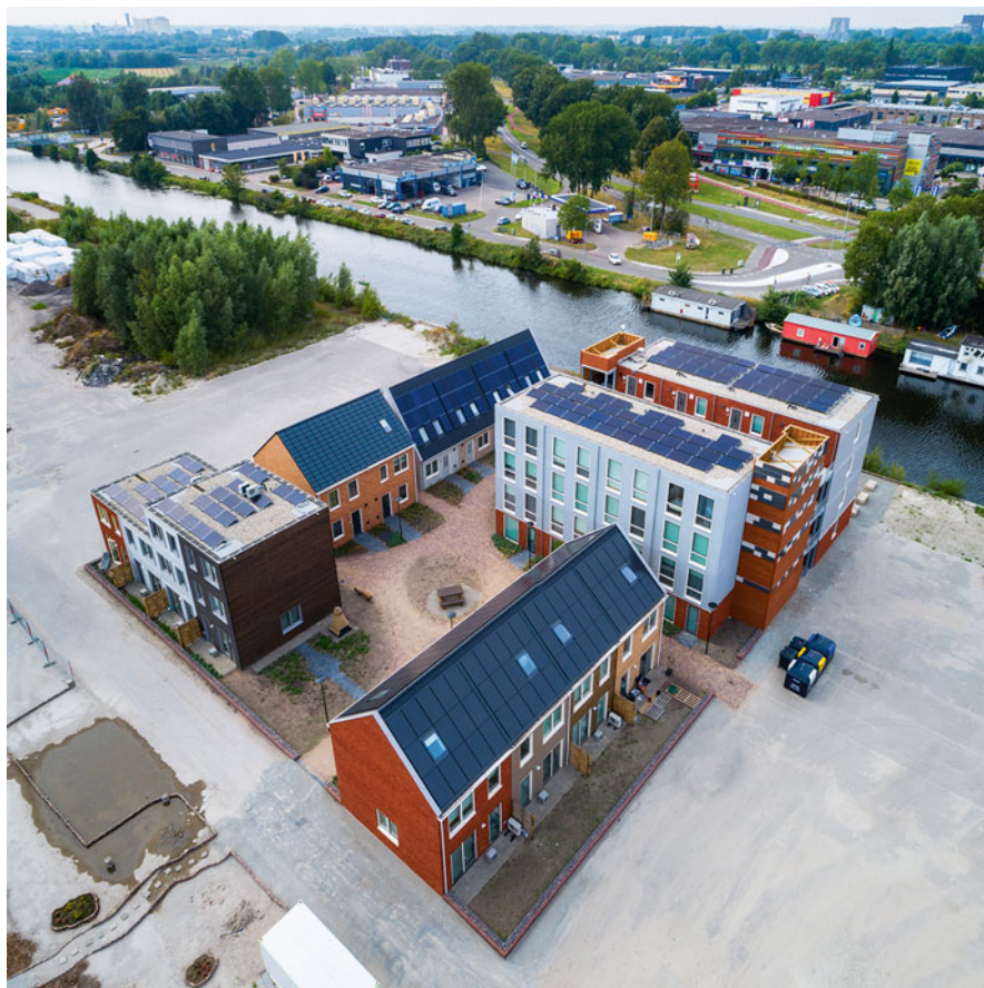
Fig. 2.6 The loading loskade just after realisation in August 2019
