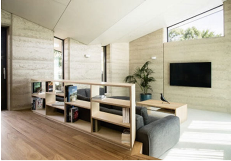
Fig. 36.3 Rammed earth walls at Passive Butterfly. (Photography by Amorfo)
