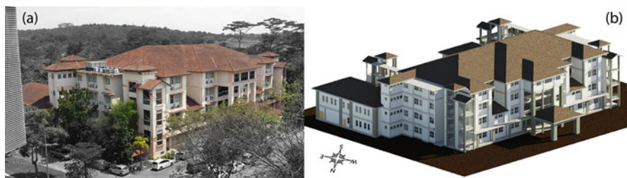
Fig. 13.4 Case study building for the RBIM framework testing; (a): photo, (b): BIM model
