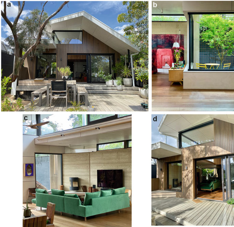
Fig. 36.7 (a) Terraced Deck conceals 11,000 l of rainwater storage supplying irrigation, toilets and laundry. Rear garden includes permaculture productive garden; (b) Northern kitchen courtyard brings light and solar warmth – deciduous Japanese Maple provides shade in hotter months; (c) Highlight windows strategically placed to capture winter sun and provide cross flow ventilation in summer; (d) External blinds integrated into the western façade provide protection during summer. Northern high windows capture winter sun
