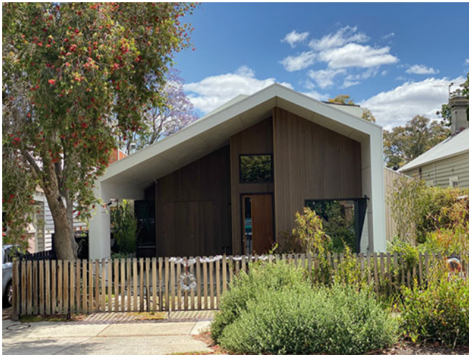
Fig. 36.6 Asymmetrical gable, inspired by local heritage homes, design to capture winter northern sun. Multi-functional entry allows home to adapt over time
