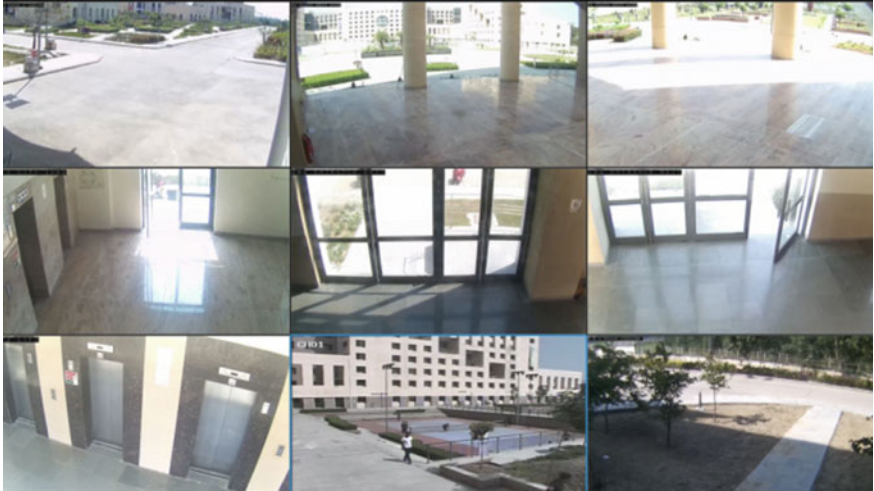
Fig. 7 CCTV monitoring of indoor locations at RG IPT to find fire or smoke
