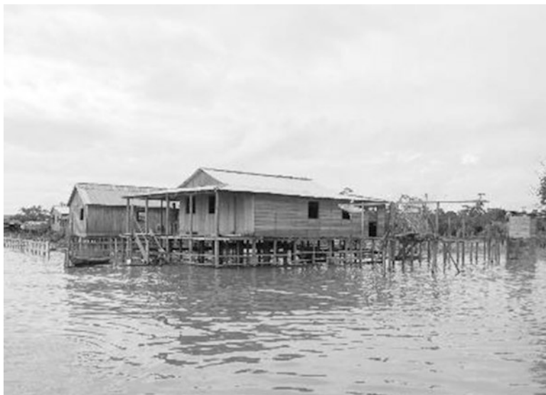
Fig. 7.10 Stilt houses in Piedade in the flooding season (March 2013). The nearest house in the photo was rebuilt one meter higher after the 2012 flood. (Photograph by E. Katz)
